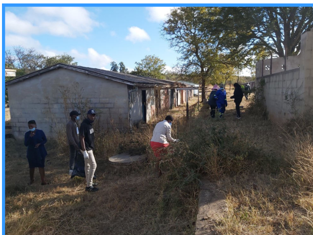
Staff members cleaning near houses under renovation to increase students and staff accommodation
